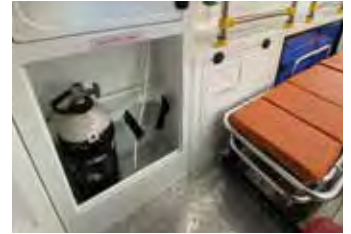
OXYGEN TANK COMPARTMENT
